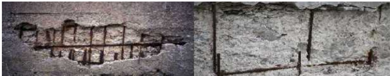
F-34 Corrosion in R.C.C structure
