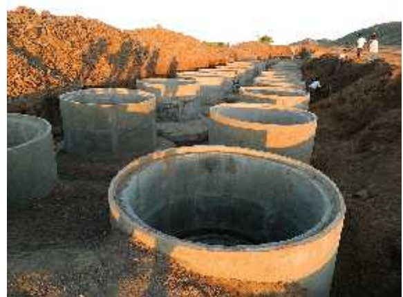
F-6 Common Biogas Plant Payvihir
