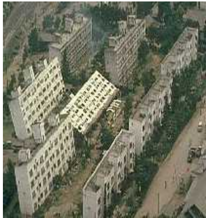
F-30 Effects of Soil liquefaction
